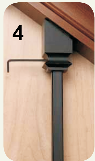
4 Slide Shoe In Place And Tighten
